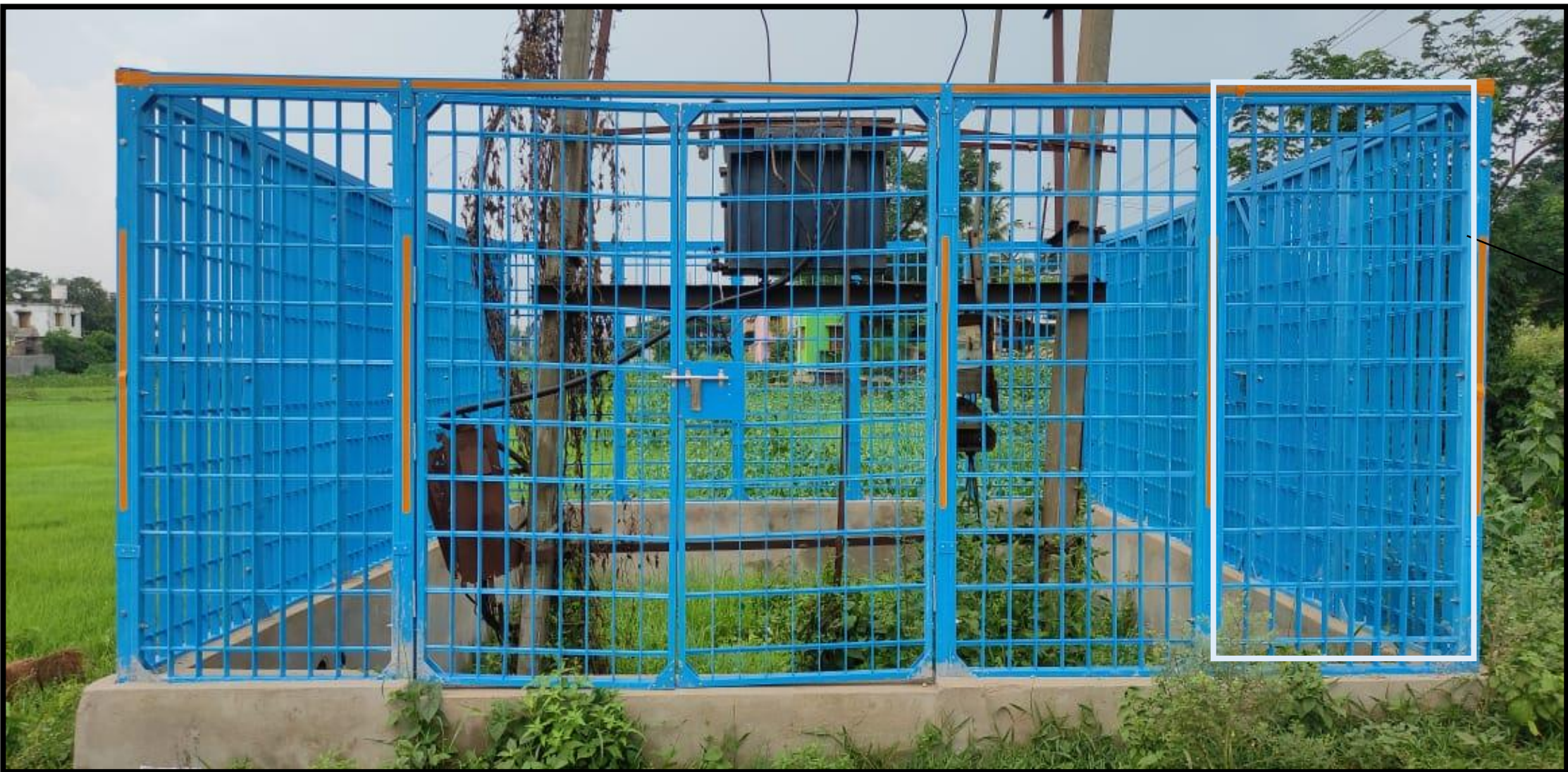
Complete FRP Fencing along with Toe wall and other accessories
